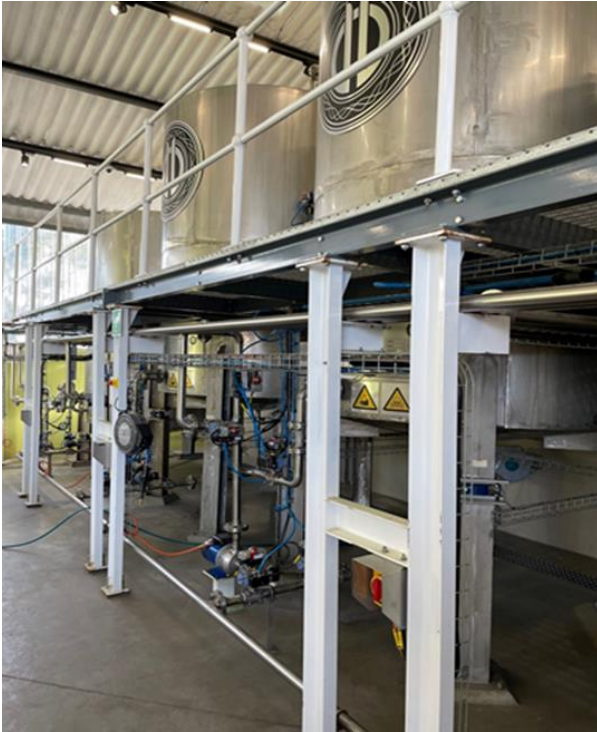
Figure 5.3: Bulk storage of CCA and delivery in bulk or kegs.
