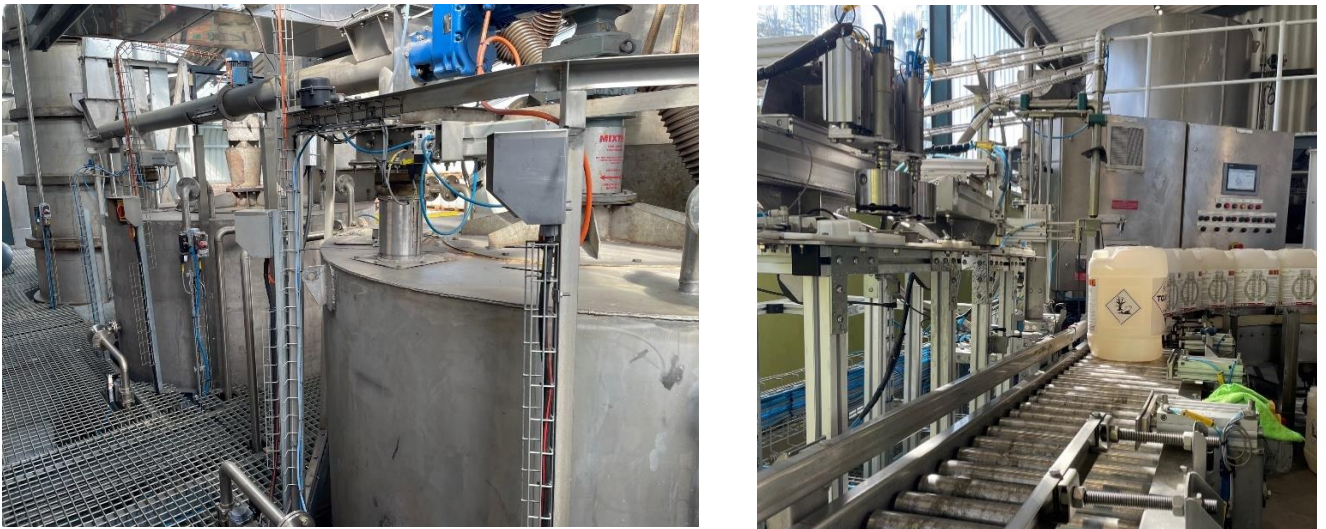
Figure 5.2: Photograph of the production reactors and the packaging line.
